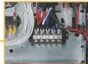
Outdoor unit power supply terminal block
