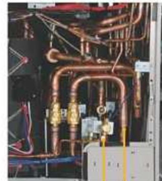
Liquid pipe Gas pipe
